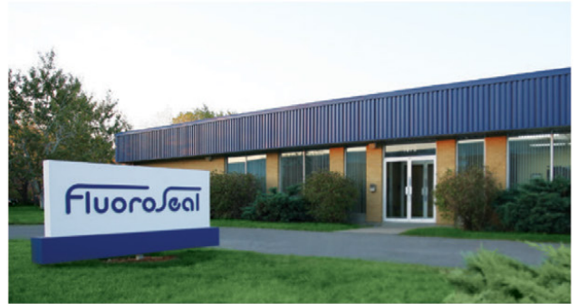
Headquarters & Foundry - Lachine, QC, Canada
